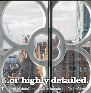
The level of detail on a wall or façade is often referred to as articulation - this term is used to describe the level of complexity on a surface. Casting precast concrete in carefully constructed moulds means that very highly articulated panels can be made.
