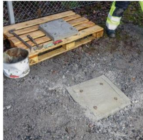
FIGURE 6 REMOVED GROUT PAD AND EXPOSED FOUNDATION WITH COPRA® ANCHORING COUPLERS
