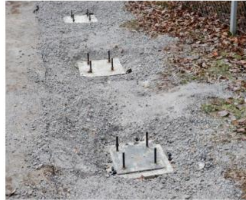
FIGURE 4 FOUNDATION WITH HPM® ANCHOR BOLTS FURTHER BACK AND FOUNDATION WITH COPRA® ANCHORING COUPLERS IN THE FOREFRONT
