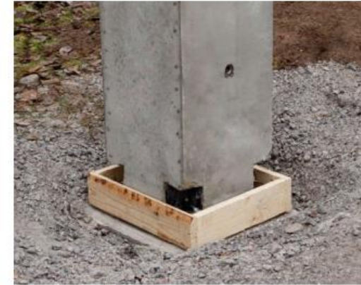
FIGURE 5 PRECAST COLUMN INSTALLED ON A FOUNDATION WITH TIMBER FORMWORK
