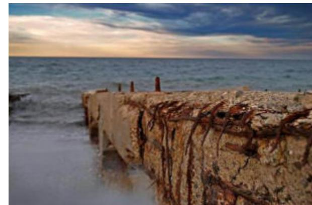
**To determinate the advance of chlorides ions inside the concrete as function of time, we can use the following expression, based on the 2<sup>g</sup> Fick´s diffusion law:**
