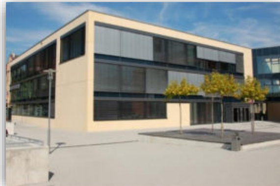
Alfons-Kern-School, Pforzheim (Germany)
