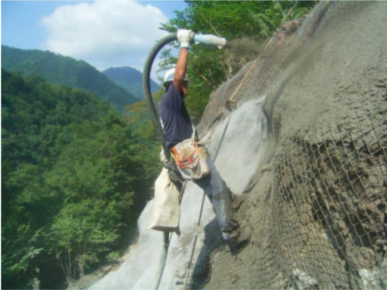
Slope Reinforcement by Shotcrete
